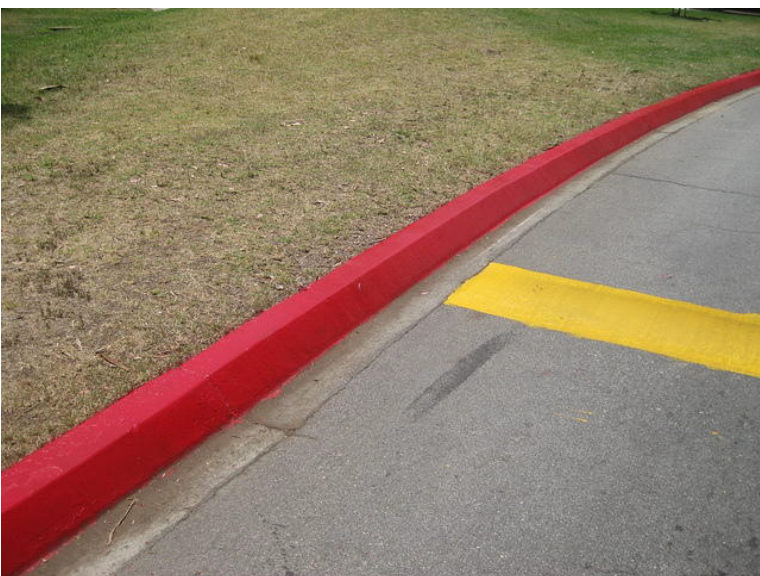
A view of one of the speed bumps right next to a freshly painted curb.
